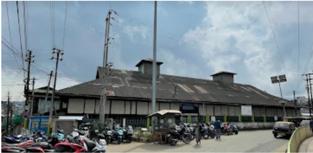
FIGURE 4: BUILDING OF INSPECTOR OF SCHOOLS FROM MAWKHAR ROAD
