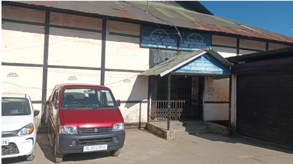
FIGURE 5: MAIN ENTRANCE GATE
